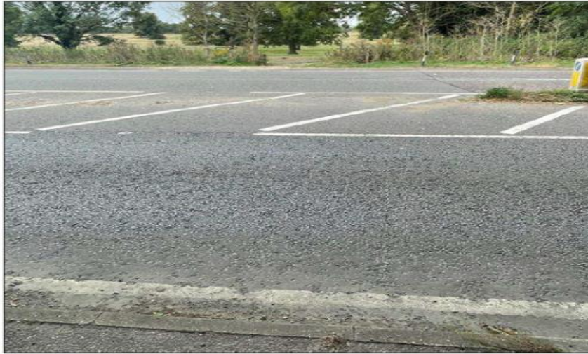
Photo 3.7 – A41 Adjacent to Future Pedestrian/Cycleway Entrance
